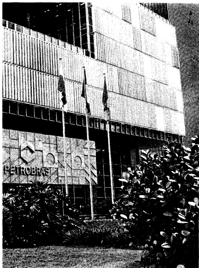
Petrobrás headquarters in Rio de Janeiro.
