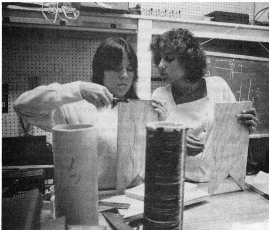
Students construct the apparatus for Ampère’s experiments. In the foreground is the solenoid—a piece of PVC pipe with copper wire coiled around it, which is needed to cancel out the effect of the Earth’s magnetic field.
