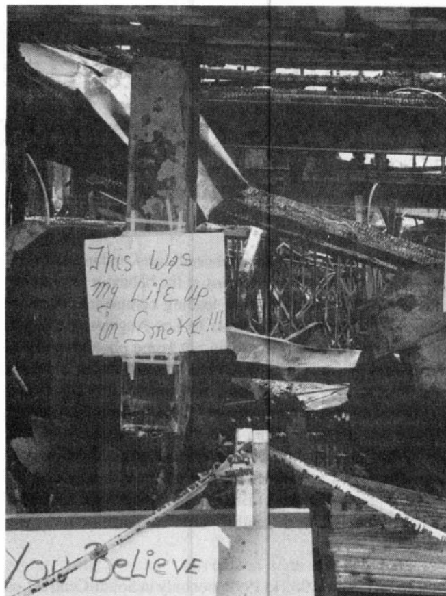
A building burned out in the Los Angeles riot—you can thank Warren Christopher, for one.
