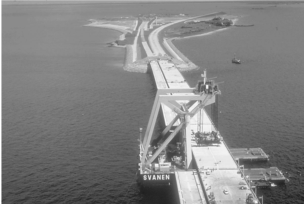
A view of construction on the West Bridge section of the Great Belt Fixed Link project. Most often, the concept of new technologies is associated with computer science, space programs, or other exotic technologies. But an often-overlooked aspect of large-scale infrastructure projects, is the development of new technologies.
