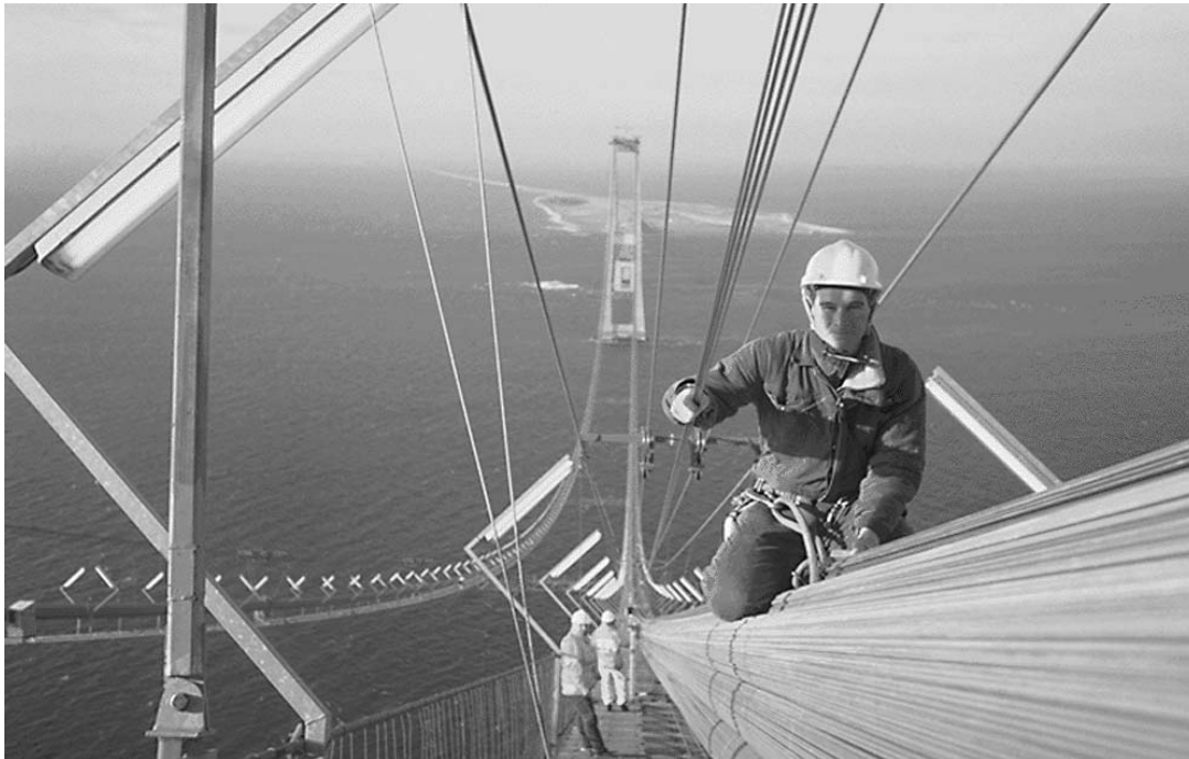
The suspension bridge under construction.
