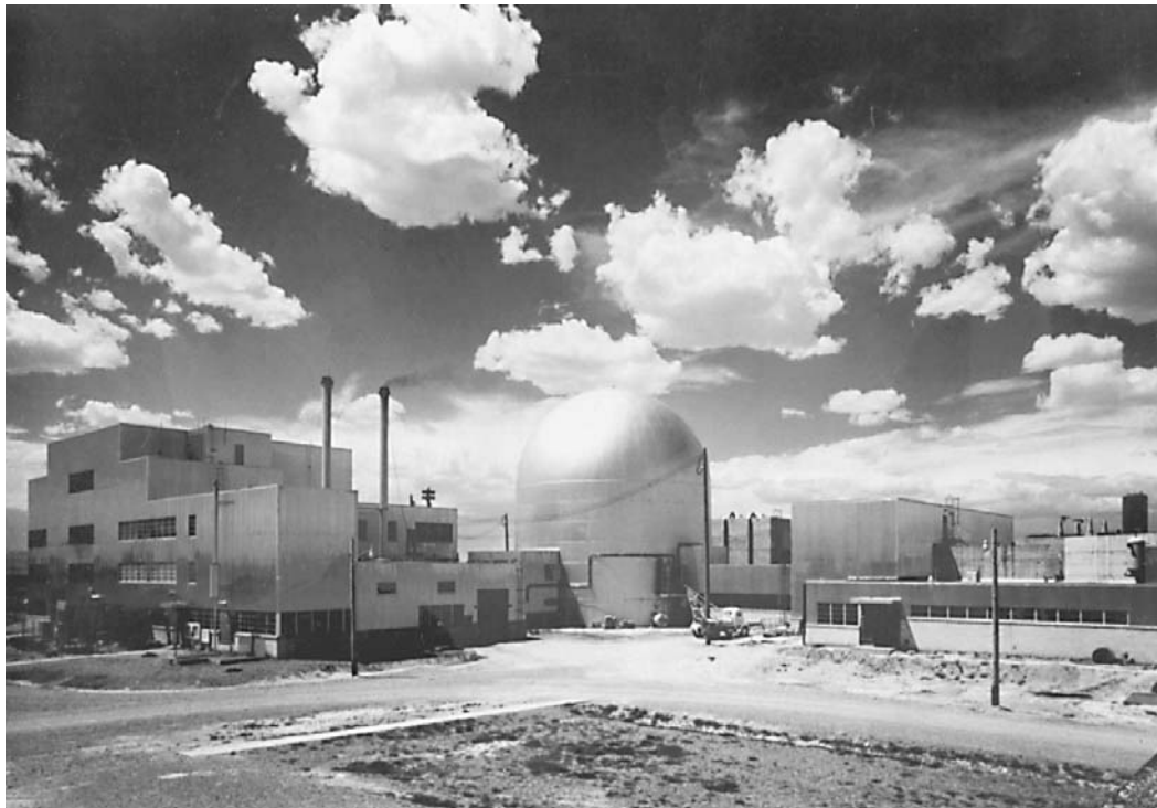
EBR-II, the experimental breeder Reactor No. 2, at Argonne National Laboratory West, operated successfully from 1964 to 1994. It was a pool-type breeder, with a passive safety system, and Argonne called it “the most successful test reactor ever.”
