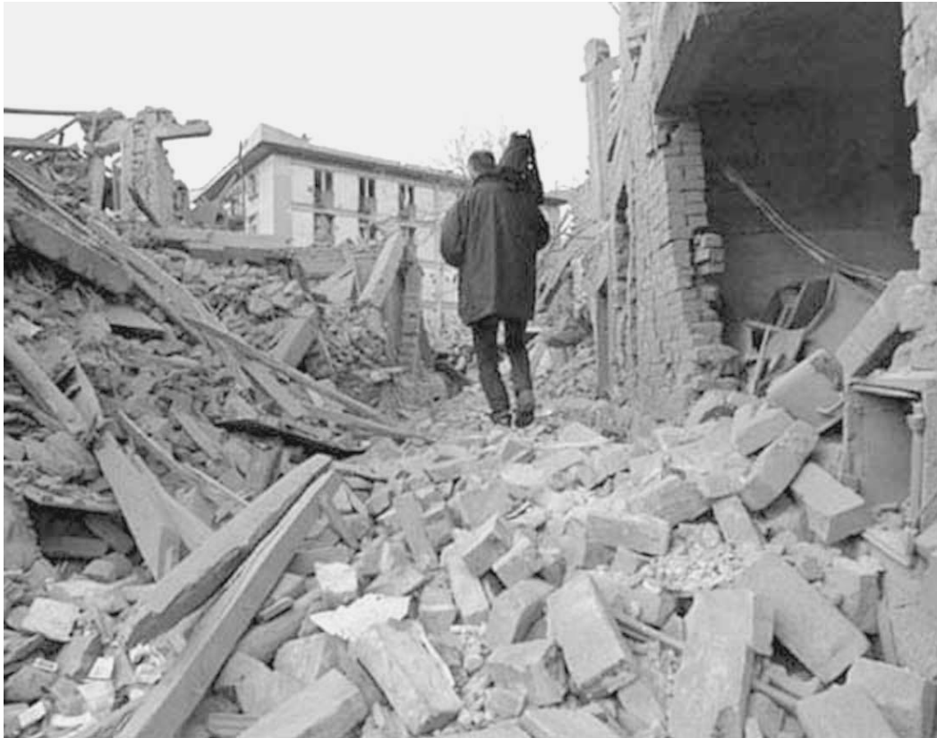
Devastation in Aleksinac, Yugoslavia, May 1999. The Balkan countries need a real "Marshall Plan" of reconstruction, not the kind of penny-pinching fraud that was perpetrated against Bosnia by the International Monetary Fund and World Bank.
