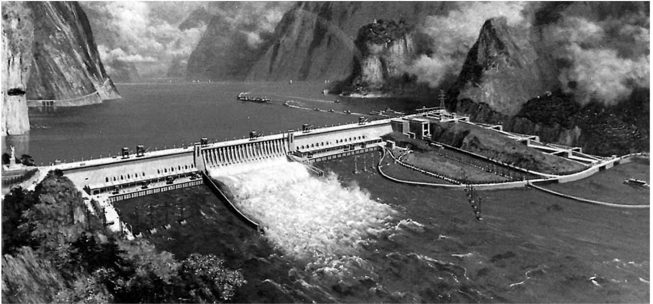
Artist's representation of China's Three Gorges Dam project. "Large-scale construction programs in infrastructure are the most natural rapid stimulant of levels of employment and of all other economic activity, in the region where such infrastructural developments are operating. The impact of the U.S.A. TVA, and a comparison of the TVA with China's ongoing Three Gorges Dam project, is a suitable illustration."
