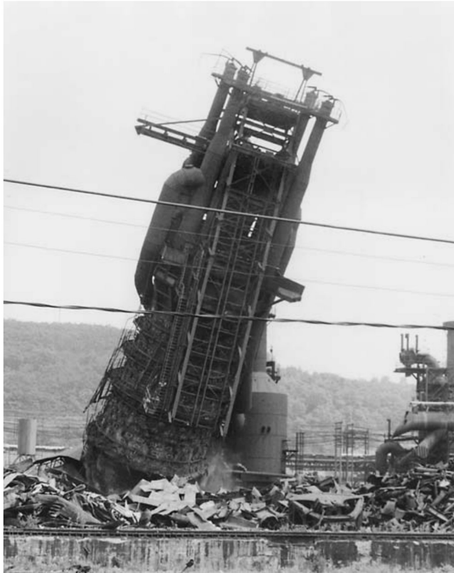
Demolition of a U.S. Steel plant in McKeesport, Pennsylvania, 1985. It is this “rust belt” phenomenon, which typifies the developments which have made the U.S. economy so vulnerable to the crisis of the region including California, today.
