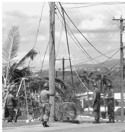
Repairing downed power lines.
