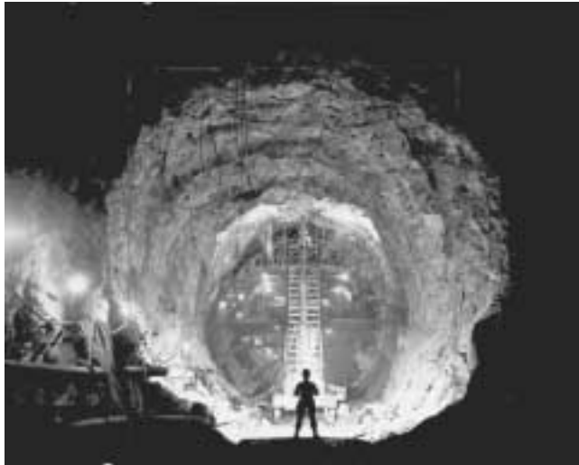
The Snowy Mountain Scheme's underground power station Tumut 1, under construction in 1958.
