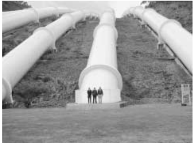
The six pipes of power station Tumut 3 are each 487 meters long, 5.6 meters in diameter, and collectively contain 10,260 tons of steel.
