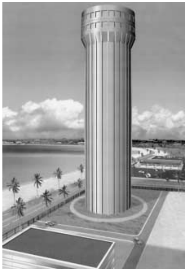
Artist's depiction of a modern seawater desalination tower. It is proposed for a location on the Pacific Coast of California. The structure houses a multi-effect distillation process (vertically stacked evaporators) for large-scale output (284,000 cubic meters daily).
