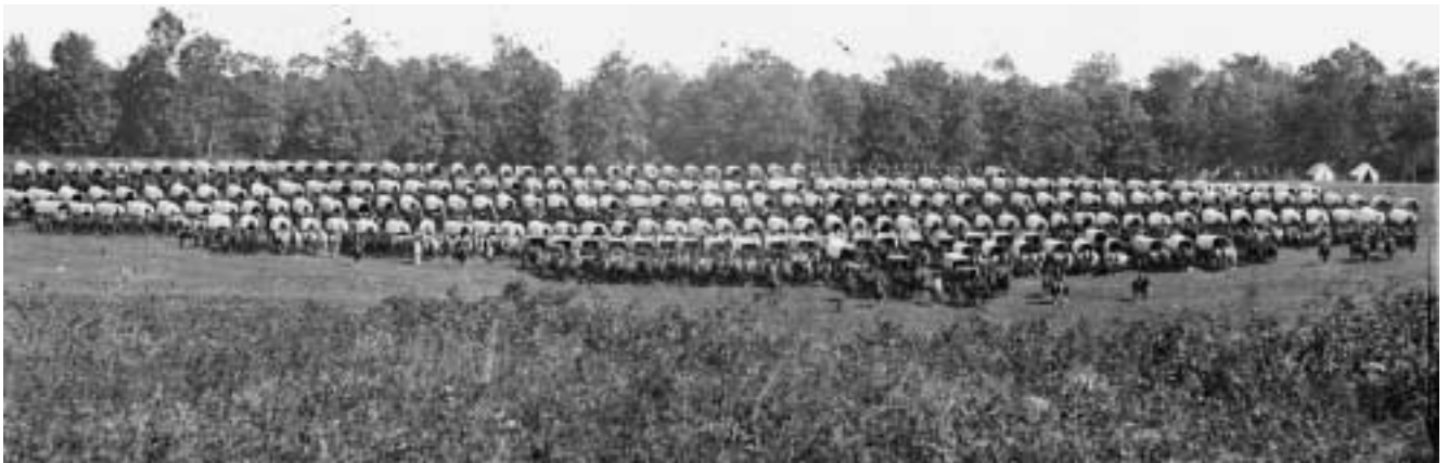
In May 1864, some 4,300 supply wagons followed the Union Army as it moved south to The Wilderness battlefield in Virginia. Creating the massive infrastructure required to sustain the troops, who were fighting deep in enemy country, was one of the colossal achievements that made victory possible.
