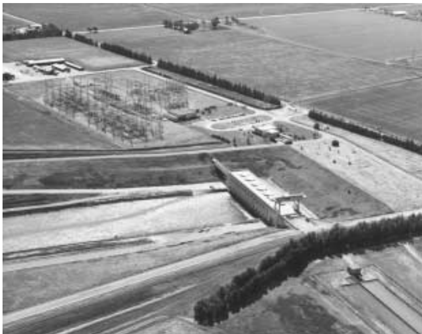
The Tracy Pumping Plant near Tracy, California, lifts water to the dry San Joaquin Valley. Water infrastructure development programs, a "NAWAPA-Plus," can make the Great American Desert bloom as well, in the interests of both the United States and Mexico.
