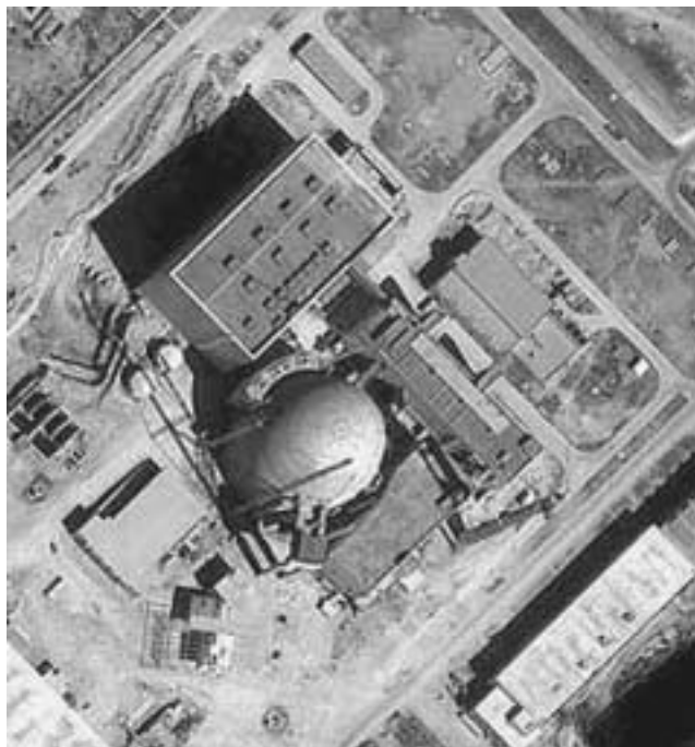
Iran's Bushehr nuclear reactor, under construction with Russian assistance. Contrary to the claims of U.S. neo-cons who know nothing about physics, it is no easy matter to extract plutonium from the spent fuel in the power plant for weapons purposes.
