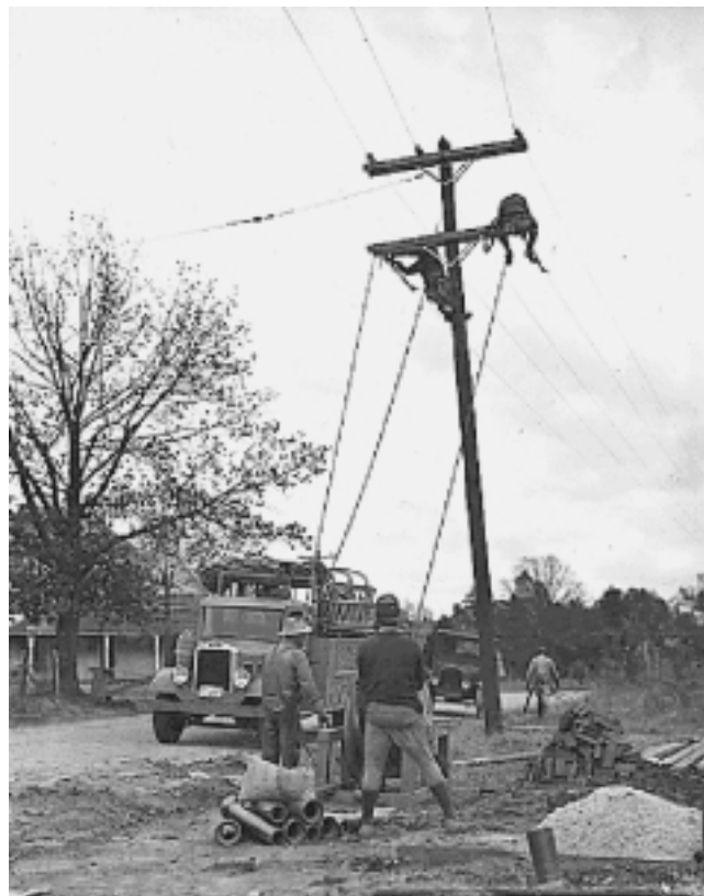
Franklin Roosevelt's Rural Electrification Act had incomparable effects on the productivity of U.S. agriculture. This shows electrical wire being strung in rural areas where the TVA was producing power.
