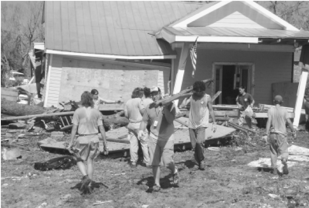
AmeriCorps members clear debris from a house in Pass Christian, Miss. in September 2005, following Hurricane Katrina. The AmeriCorps is not being used effectively, LaRouche said, but can be upgraded to undertake new missions, as we retool the auto industry.
