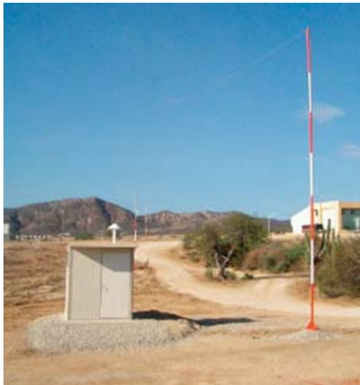
b) An example of the installation used
