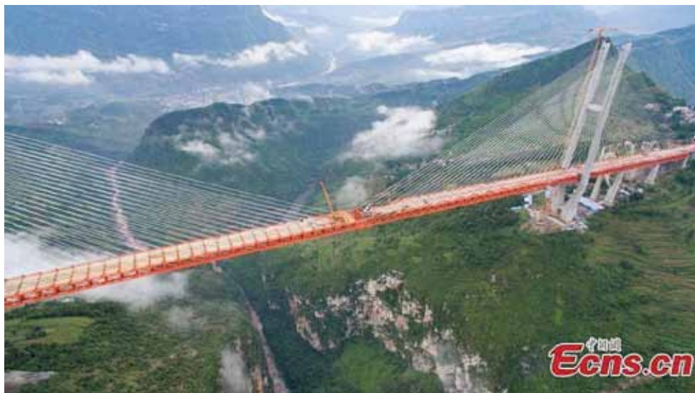
China News Service/Pan Xianyang World's highest bridge, the Beipan River expressway bridge—part of a highway linking the cities of Hangzhou and Ruili—opened Dec. 29, 2016.
