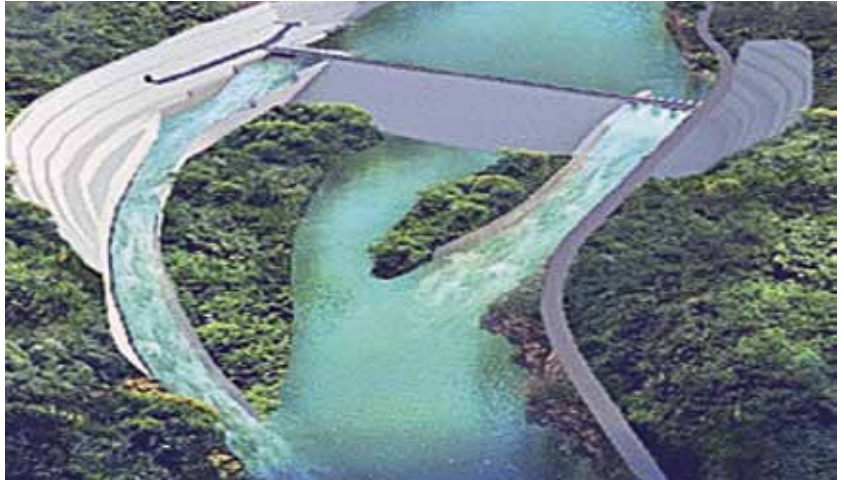
Suki Kanari hydropower station under construction, another project of the China-Pakistan Economic Corridor in Pakistan.
