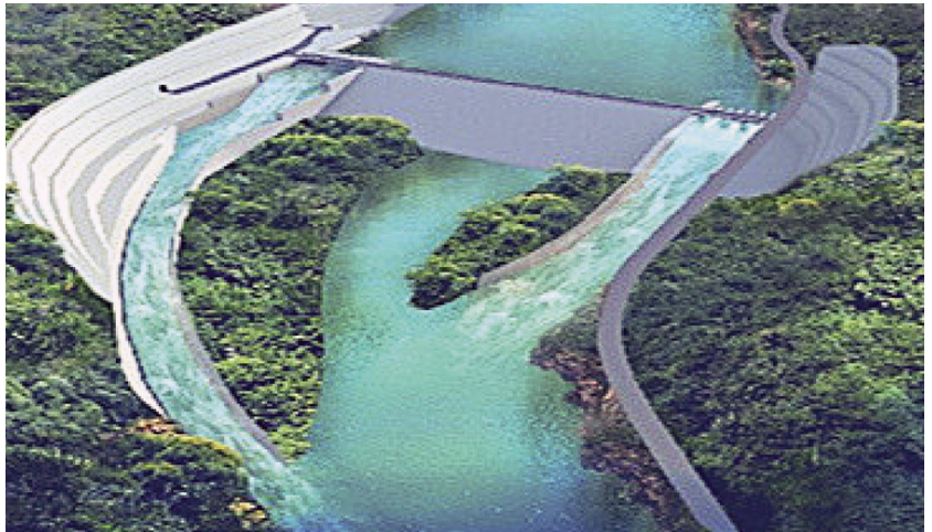
Suki Kanari hydropower station under construction, another project of the China-Pakistan Economic Corridor in Pakistan.
