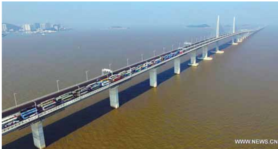
The just completed, 55-km Hong Kong-Zhuhai-Macao Bridge connects the three cities on the Pearl River Delta.
