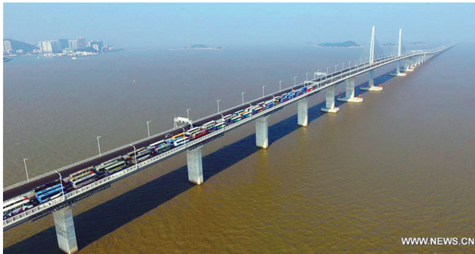
The just completed, 55-km Hong Kong-Zhuhai-Macao Bridge connects the three cities on the Pearl River Delta.
