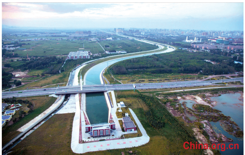
The exit of the Qilihe Canal Inverted Siphon Project.
