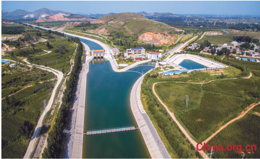
The Xiheishan flow division gate.
