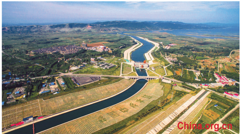
The head of the middle route of the South-North Water Diversion Project.
