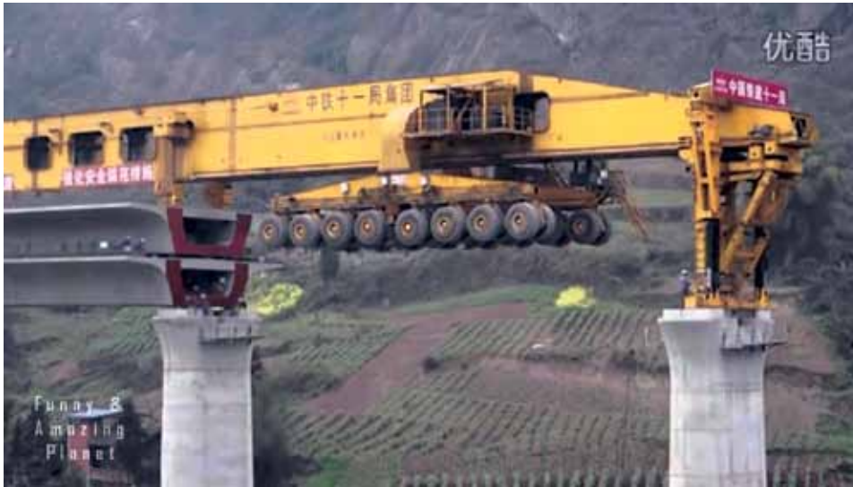
Machine in China enabling rapid placement of elevated trestles.
