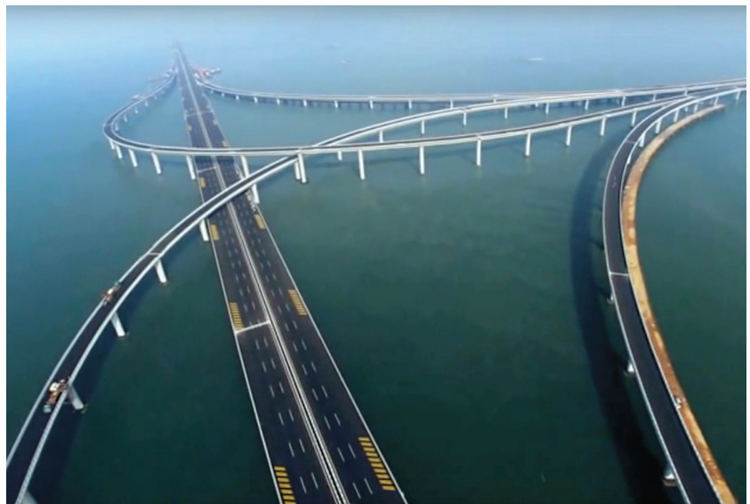
Danyang-Kunshan Grand Bridge in China.
