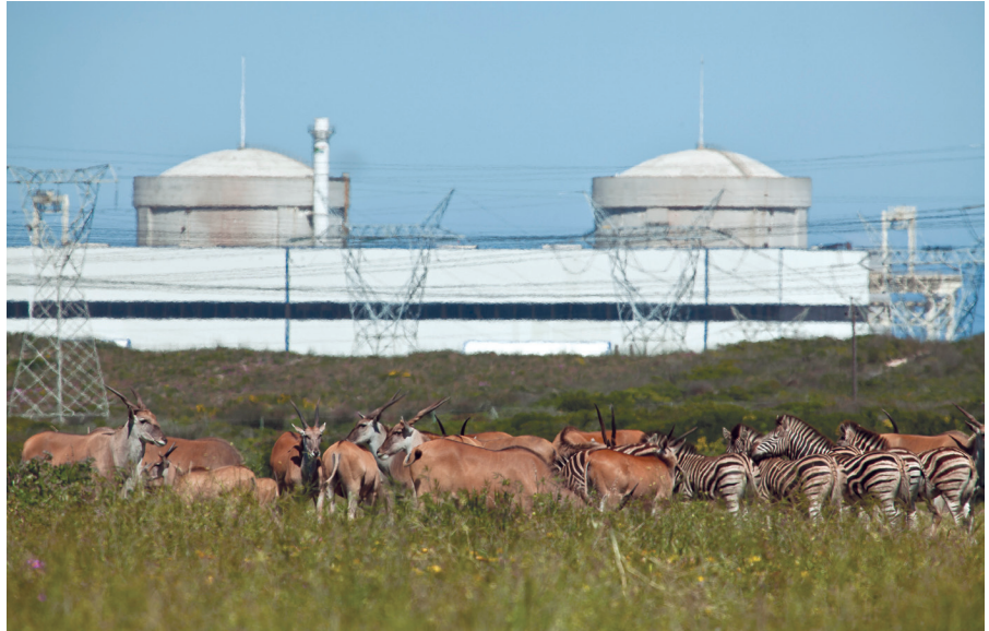
The Koeberg nuclear power plant, 30 km north of Cape Town, South Africa. The plant, which includes two pressurized water reactors running on enriched uranium, is rated at 1,860 MW. It is owned and operated by the state-owned electricity corporation, ESKOM.
