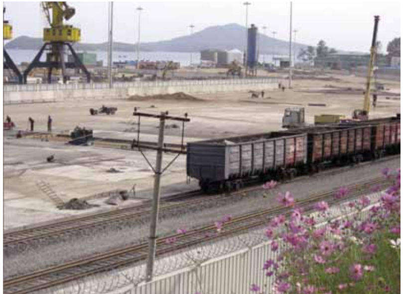
The Rason-Russia railway link, constructed by North and South Koreans along with Russians during the “Sunshine Policy” period between North and South Korea, extended a standard gauge line from Russia to Rajin Port in North Korea.
