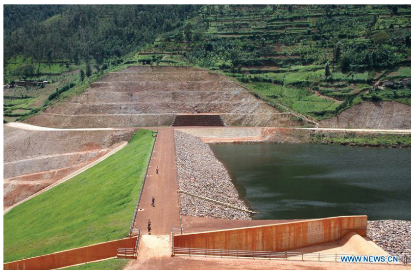
The Muzanza Dam in Rwanda, built by China Geo-Engineering Corp., Feb. 16, 2018.
