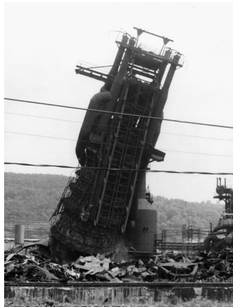
Left, demolition of an abandoned blast furnace, McKeesport, Pa., 2006. Below, homelessness in the U.S. capital, December 2010.
