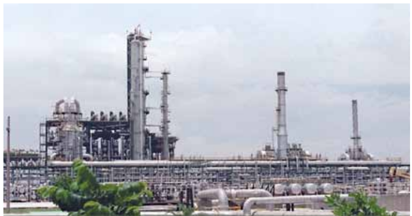
The Francisco I. Madero Refinery, owned and operated by Pemex, Ciudad Madero Tamaulipas, Mexico, August, 2017.
