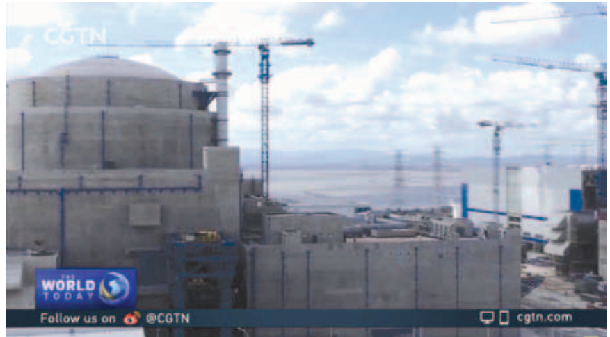
Hualong One, China's first nuclear power facility with domestically developed technology, was connected to the electrical grid on November 27, 2020.
