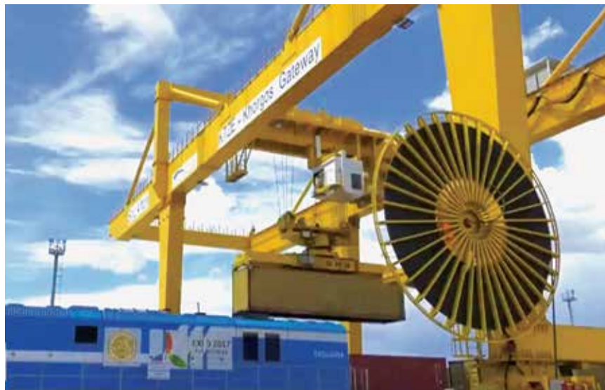
A view of the railway exchange station at the Khorgos Gateway in Kazakhstan, the largest dry port in the world, which connects Kazakhstan and China by rail. Shown, a heavy lifting crane transferring cargo between trains running on Russian Wide Gauge track and those running on Chinese Standard Gauge track.
