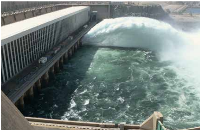
The building of the Aswan High Dam and its power plant was a priority for Egyptian President Gamal Abdel Nasser and the Free Officers' movement he led, as a step in developing the national economy. Here, a portion of the dam's power plant. The dam, opened in 1971, is on the Nile at Aswan.
